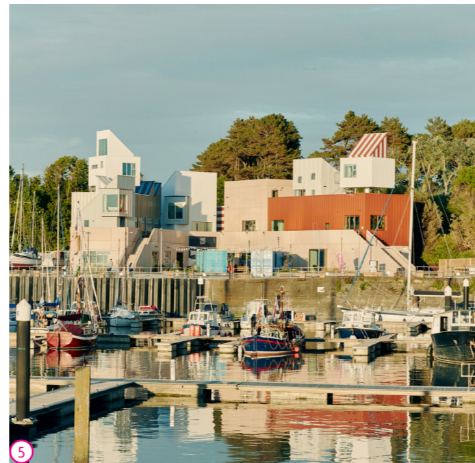
2) A jubilant community build team on completion of the pavillion at Splash Point - built by hand with 50 community volunteers over three days, bringing an overgrown unloved site back into public use.
